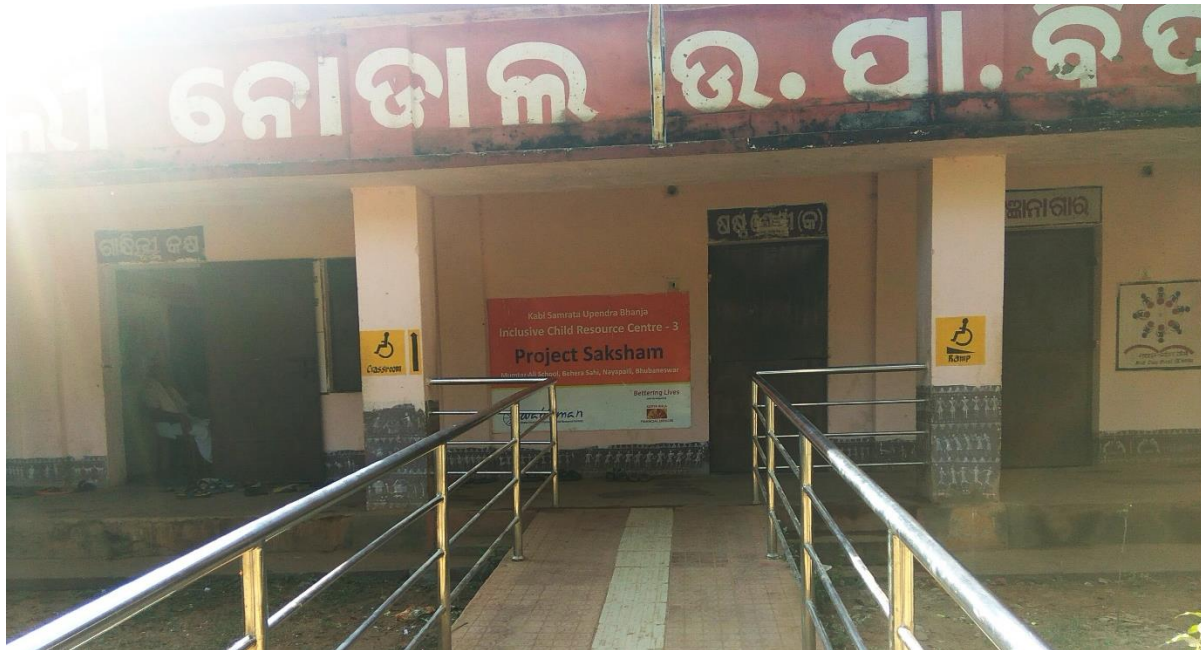
Figure 1 Ramp with railing at ICRC 3 in Mumtazalli nodal UP school
